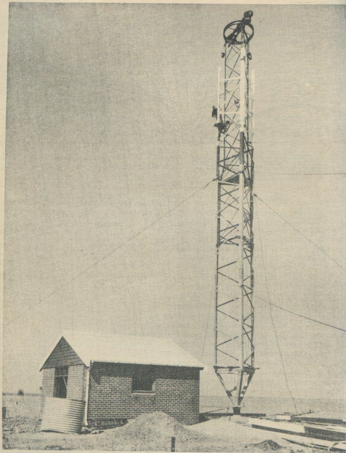
BOTTOM PART OF 3LO/AR RADIATOR. (Picture taken during erection of mast).
