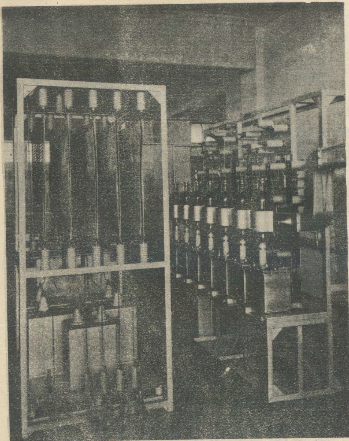
EXTRA HIGH TENSION RECTIFIER UNIT. (10 kW BROADCAST TRANSMITTER. MEDIUM WAVE.)
